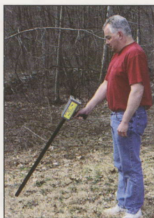
Tracking an armored cable on land
